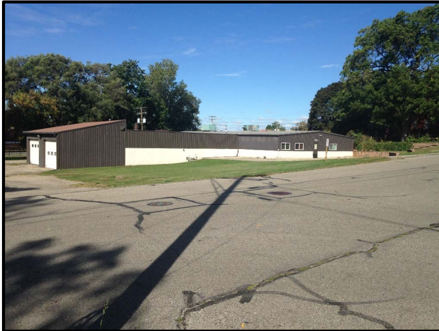
VIEW OF THE NORTHWESTERN ADJOINING PROPERTY
