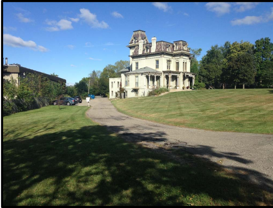
VIEW OF THE NORTHEASTERN ADJOINING PROPERTY
