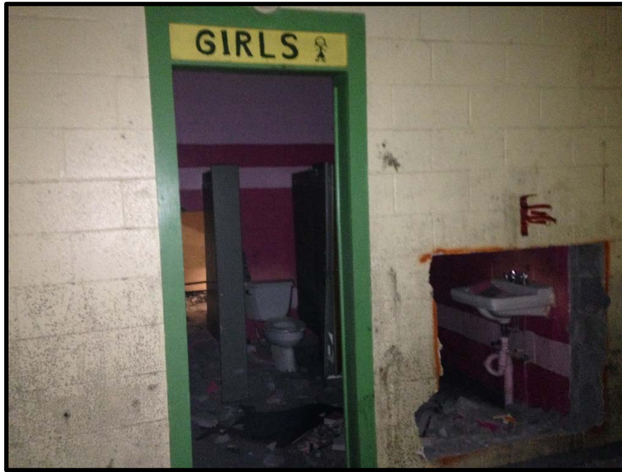
VIEW OF A TYPICAL SUBJECT PROPERTY BATHROOM
