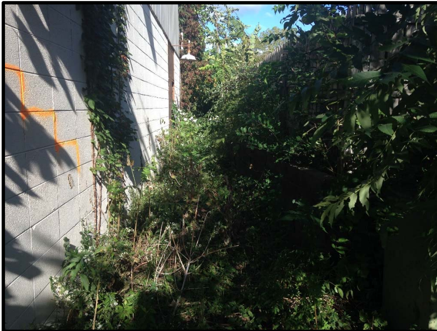
VIEW OF THE EASTERN EXTERIOR SIDE OF THE SUBJECT BUILDING
