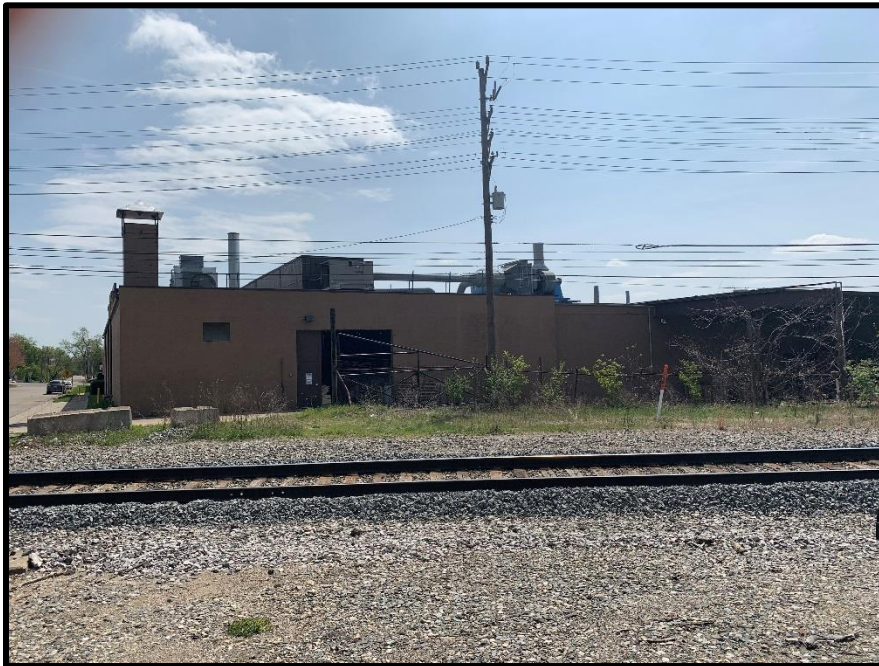
SOUTHERN ADJOINING PROPERTY (103 N. GROVE STREET)
