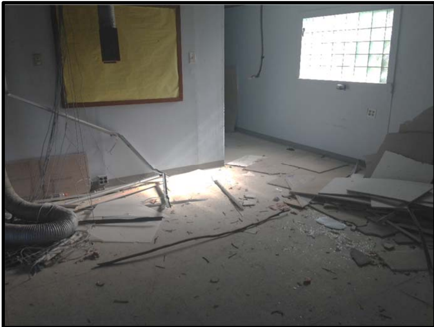
VIEW OF THE OFFICE AREA LOCATED ABOVE THE SUBJECT BUILDING GARAGE
